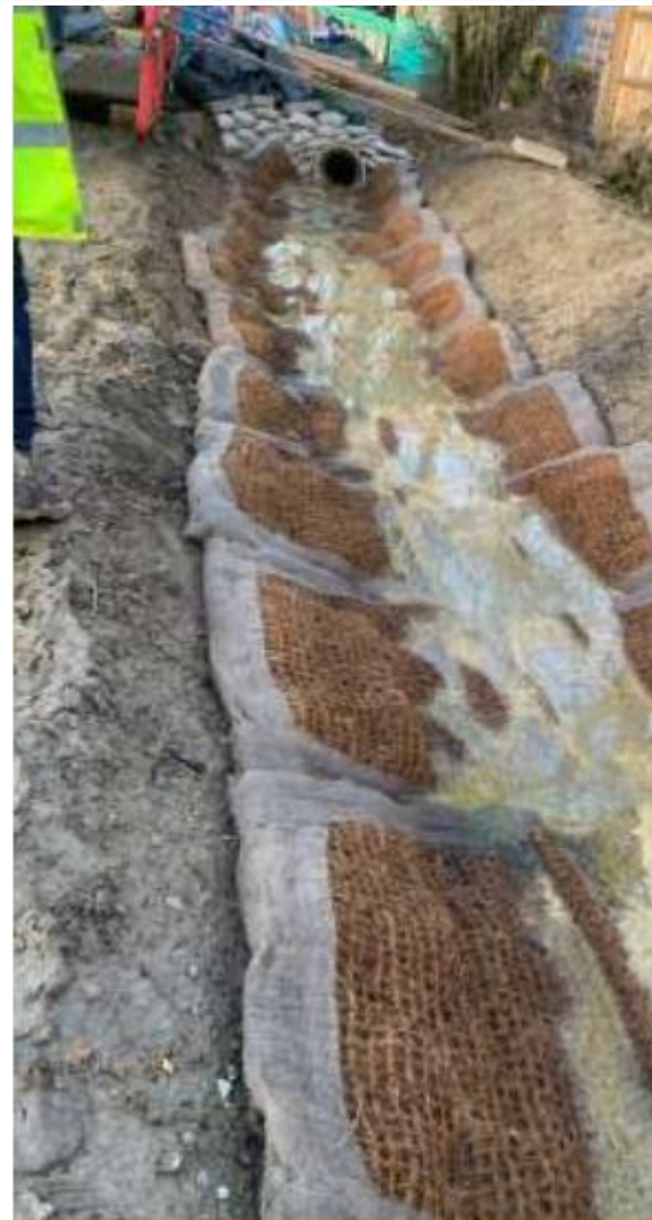
Trench with flocculant matting
